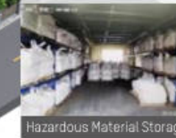
Hazardous Material Storage
